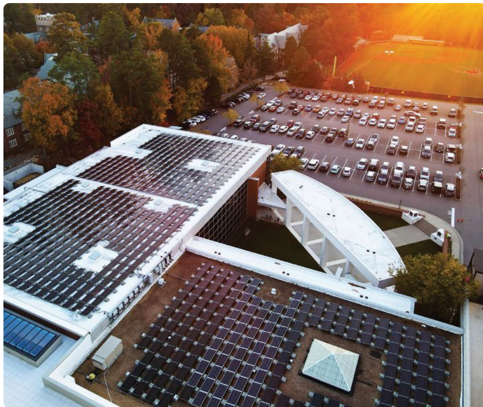
University of Richmond solar array
